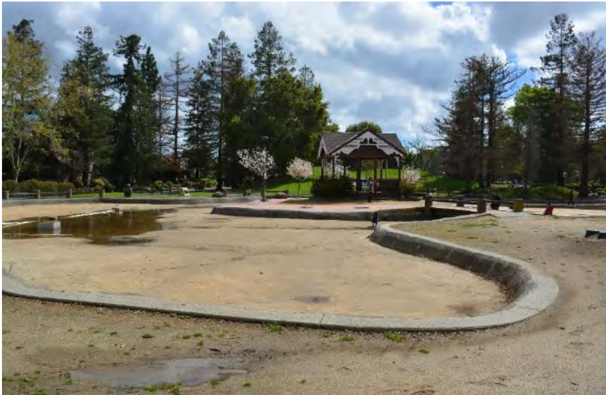
Memorial Park's gazebo and pond reflect outdated design and difficulties in adapting to changing conditions. The pond was drained during drought conditions and is not reopened.
